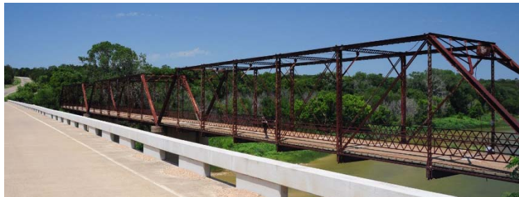
Fig. 1. Old steel truss bridge over Brazos river (www.bridgehunter.com).
