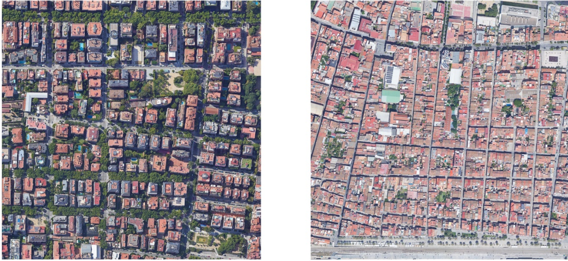
Figure 3. Aerial view of the two urban fragments selected. Tres Torres on the left, Badalona on the right (the order of presentation is maintained on the following images)
