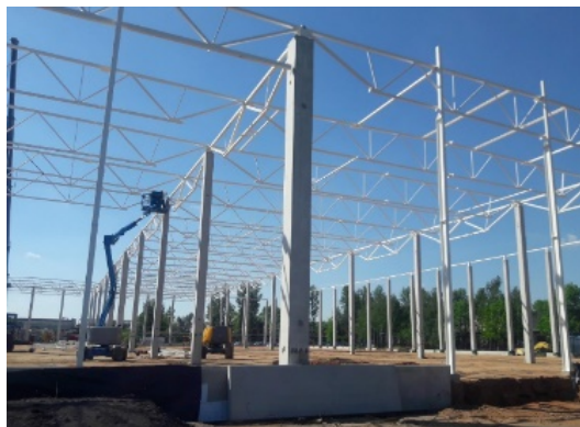
Fig. 1. Typical warehouse – construction site.
