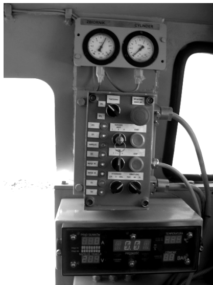
Fig. 4. Locomotive Ld-31 EM, control panel, [7]
