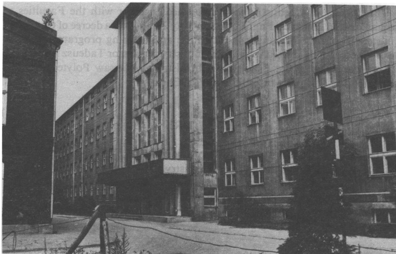
The main building of the Faculty of Chemistry
