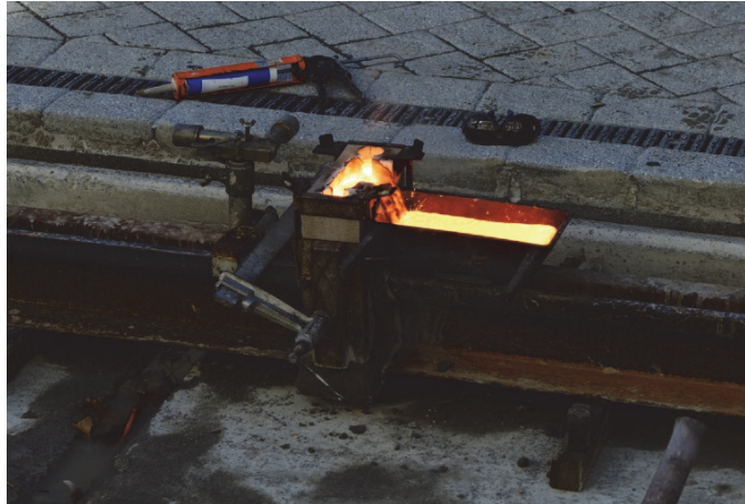
Figure 12.4. Tram tracks being joint by TW [4]
